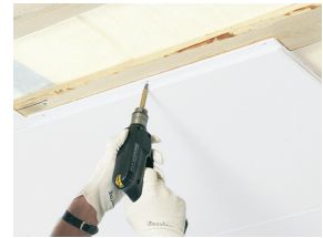
Focus F is installed by screw fixing
